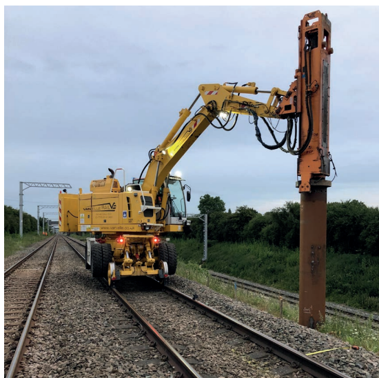
Fig. 13. Pile driving with commercially available plant
