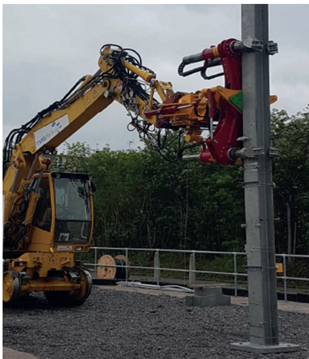
Fig 24. RRV and manipulator installing mast with pre-fixed small part steelwork
