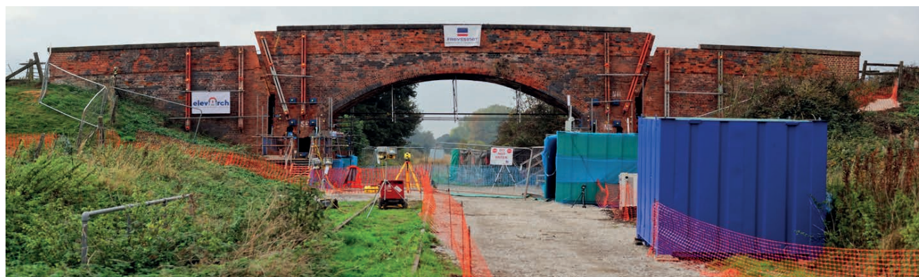
Fig. 21. The ElevArch demonstration – jacking up rather than demolishing and rebuilding a masonry arch bridge
